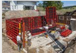
Wall Formwork
